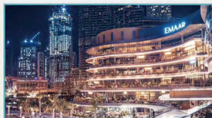
Commercial complex/municipal agency
